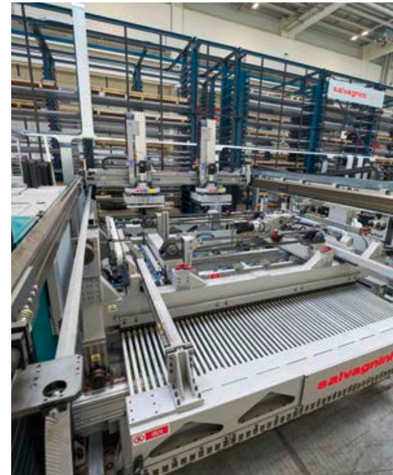
The high-bay warehouse offers 800 rack bays, from which the metal sheets are automatically collected and transported to the laser cutting unit.
