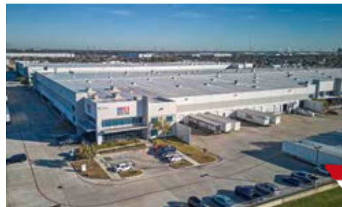
At the Rittal Application Center in Houston, customers can see the future of panel building and switchgear manufacturing for themselves and try out applications.
